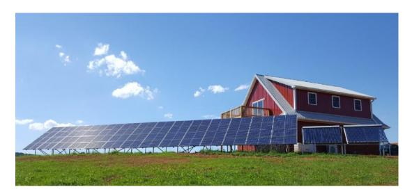
➤ The system consists of a ground mounted 16kW solar PV array with 2 grid tied SMA inverters and 2 SMA battery inverters. This system is a hybrid of solar PV, solar batteries and a back-up gas generator.
