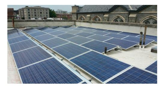
> The 34-kW solar PV system for the church has been installed using a top of the line ballasted racking system making no penetrations to the flat roof of the church.
