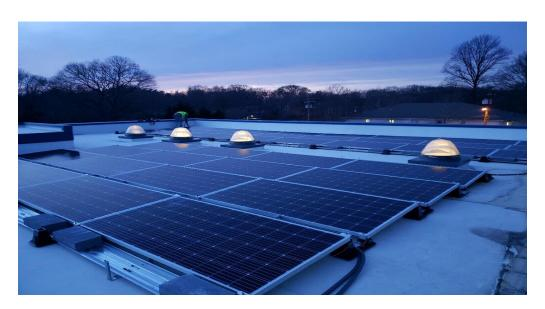
> The picture above is of a 37kW ballast-mounted PV system installed on the Anne Arundel county Eastern district polices station.
