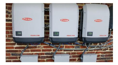
> The Engineering team at GreenBrilliance suggested installation of the newer technology based dual MPPT inverters to be used at the site which would increase the production efficiency of the system.
